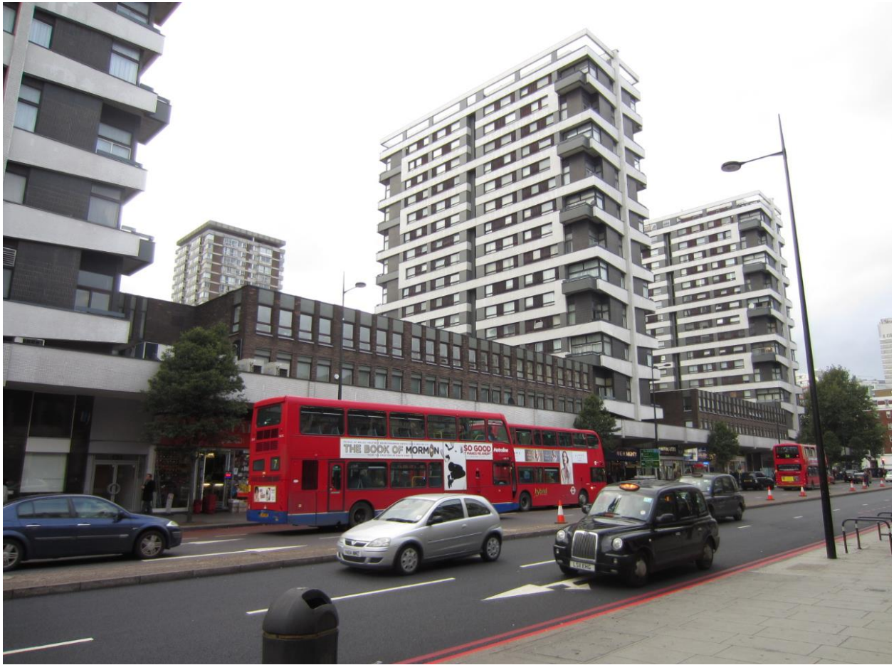
Front elevation from Edgware Road.
